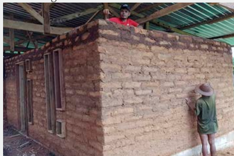
Phillipa (red) and Pah Me (green) building adobe walls.
