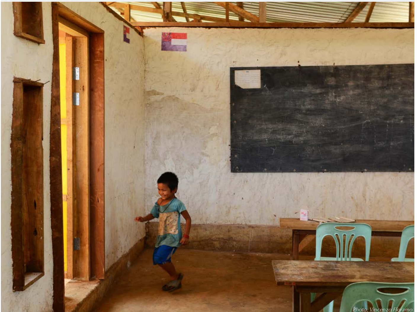
Classroom interior. The walls are given a finishing layer with limestone for longevity and a lighter impression
