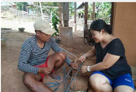
Ste Pha and Paw Eh Wah bending iron for foundation
