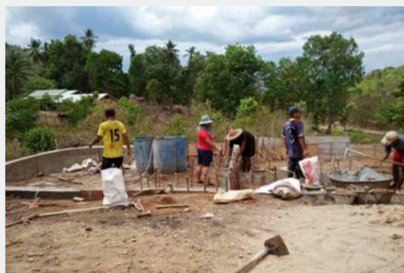
Building site - Gaw La Heh school in Je Po Kee Village
