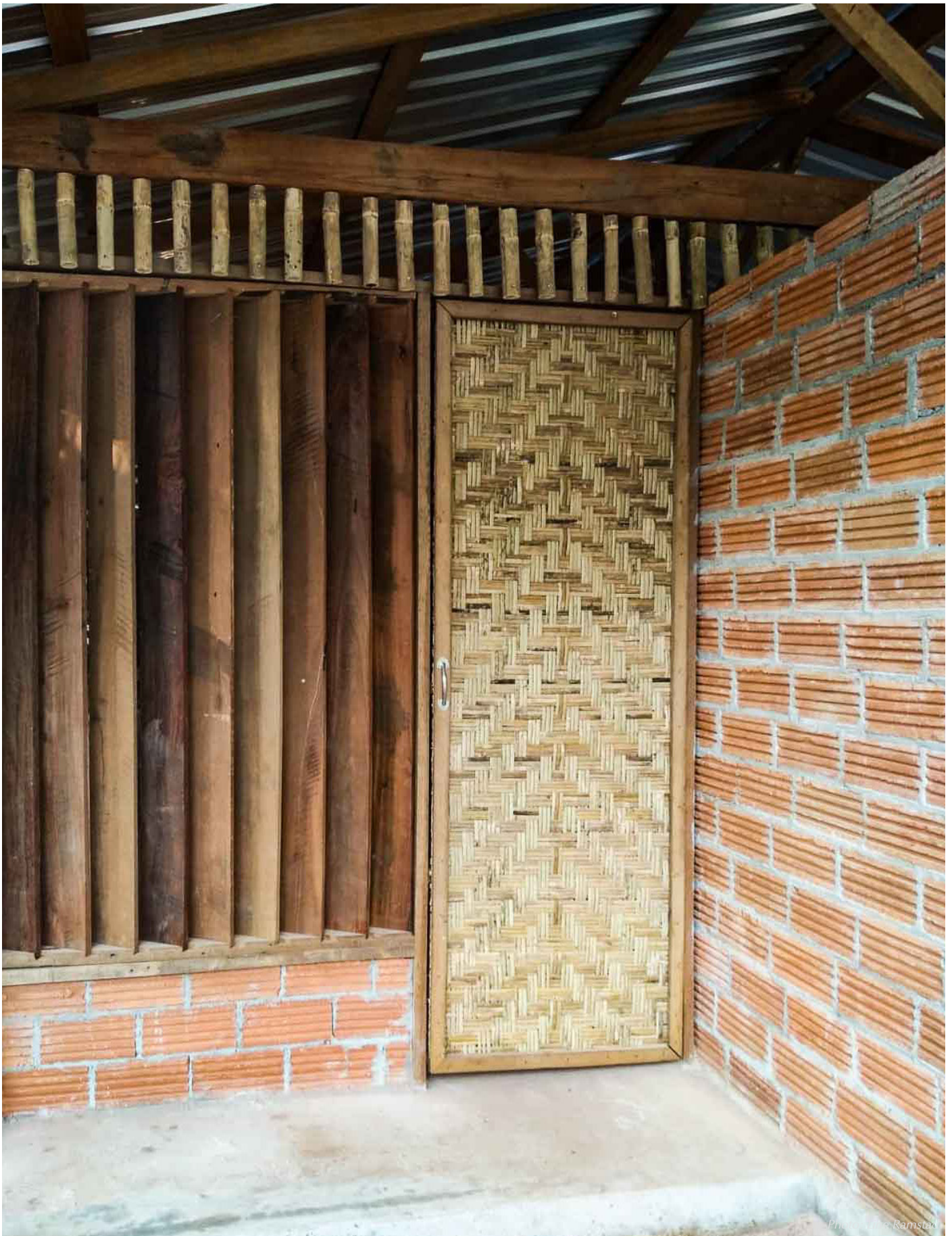
Kitchen entrance. Brick wall, window in secondhanded timber tilted to avoid direct sunlight, but get air and light through. Door with braided bamboo cover
