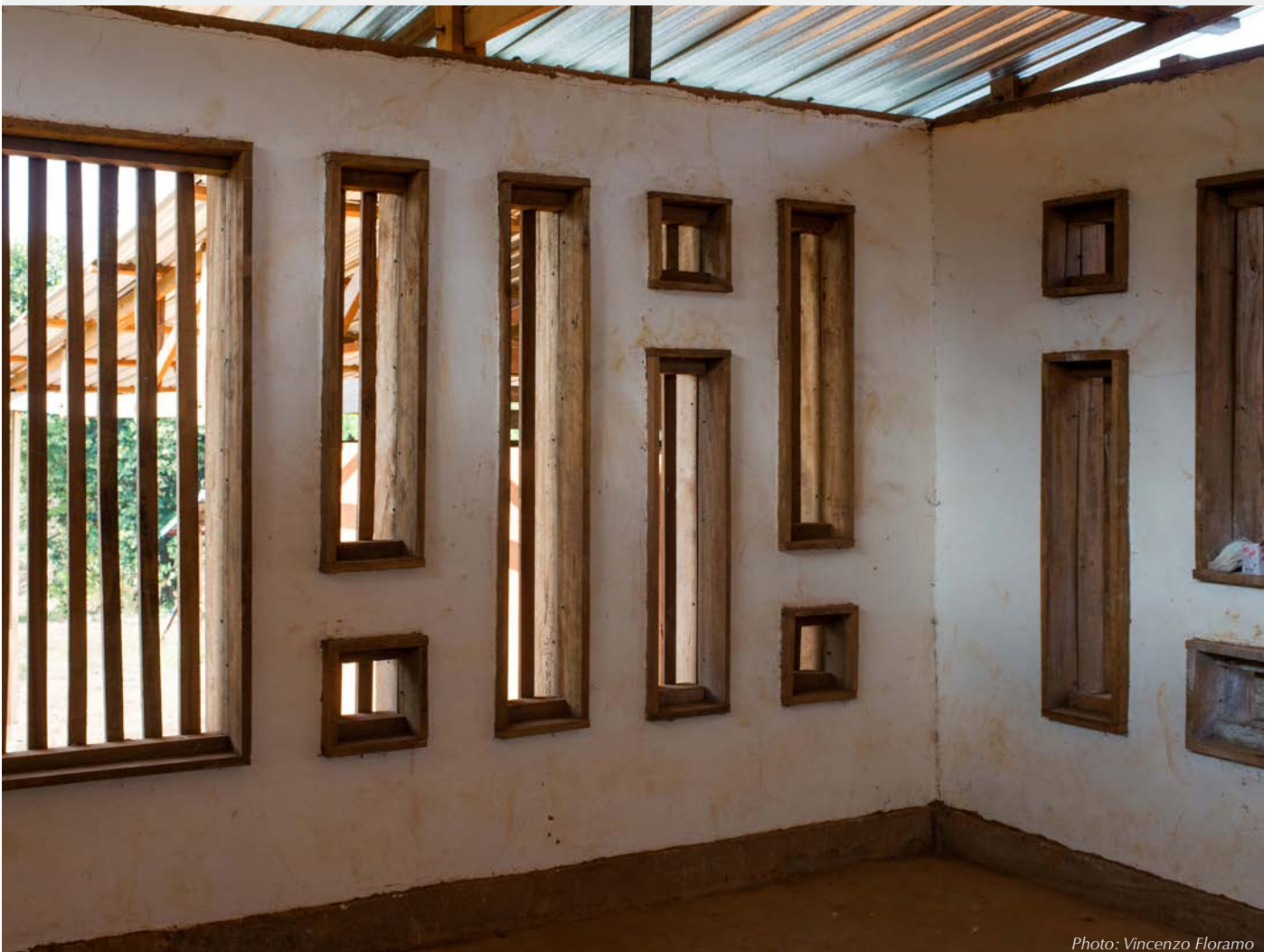
Classroom interior. Windows towards north are larger to let more daylight in, but avoid direct sunlight
